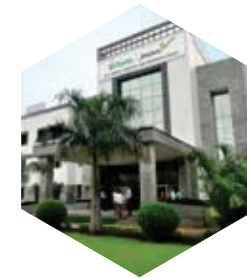
Fortis OP Jindal Hospital & Research Centre, Raigarh, Chhattisgarh
