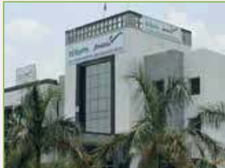
Fortis Hospital, Raigarh
